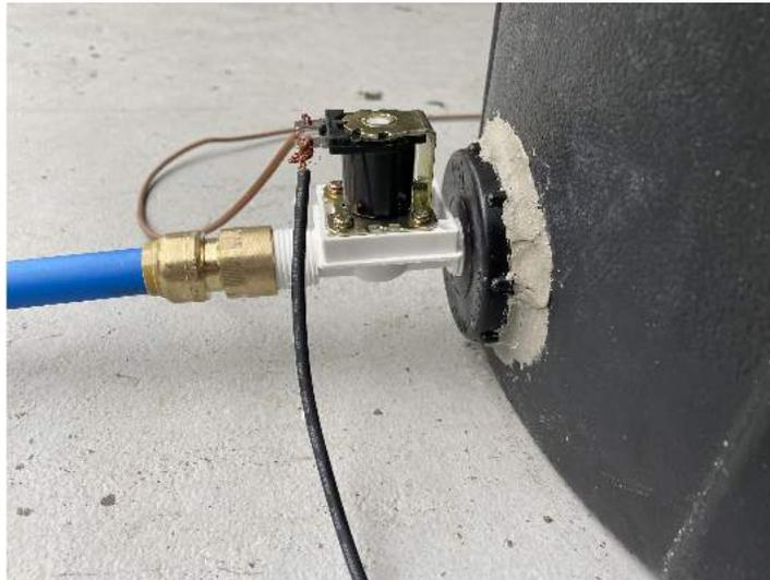
4. Then use the  $\frac{1}{2}$  pipe thread tape around both ends of the valve. Make sure the valve is nice and tight to prevent any water leaks. Make sure your valve is pointing in the direction of the water flow. These valves are unidirectional, meaning the water could only flow in only one direction. You can figure out the direction by looking at the top of the valve. There will be an arrow that points in the direction of the water flow.
